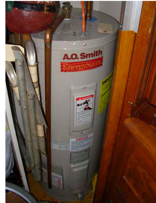
20. DHW tanks, some located in closets, others under cabinets
