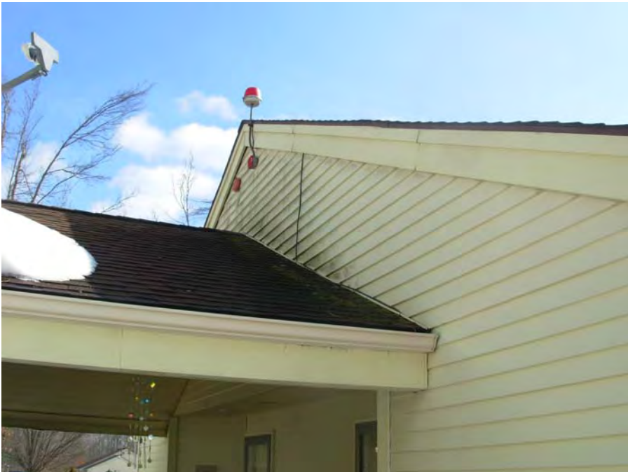
7. Organic material growth on siding and roofing shingles
