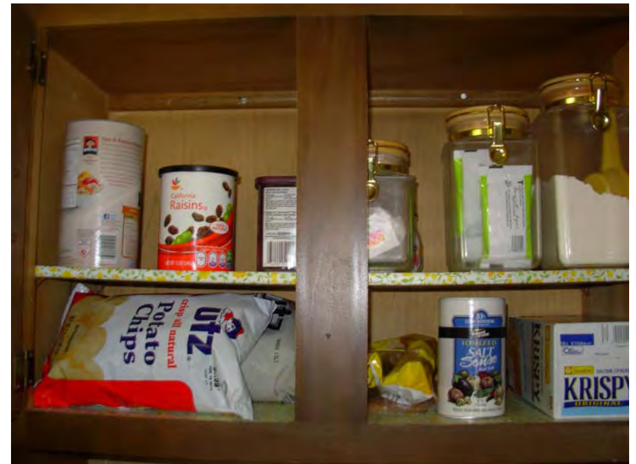
16. Sagging shelving at original wall cabinets
