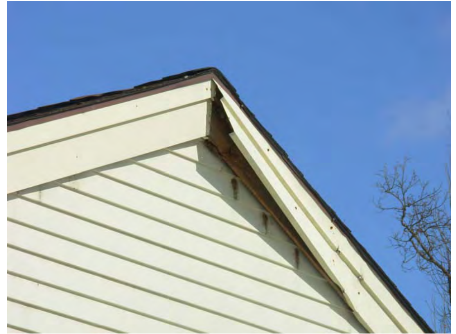
6. Spot siding and trim damage
