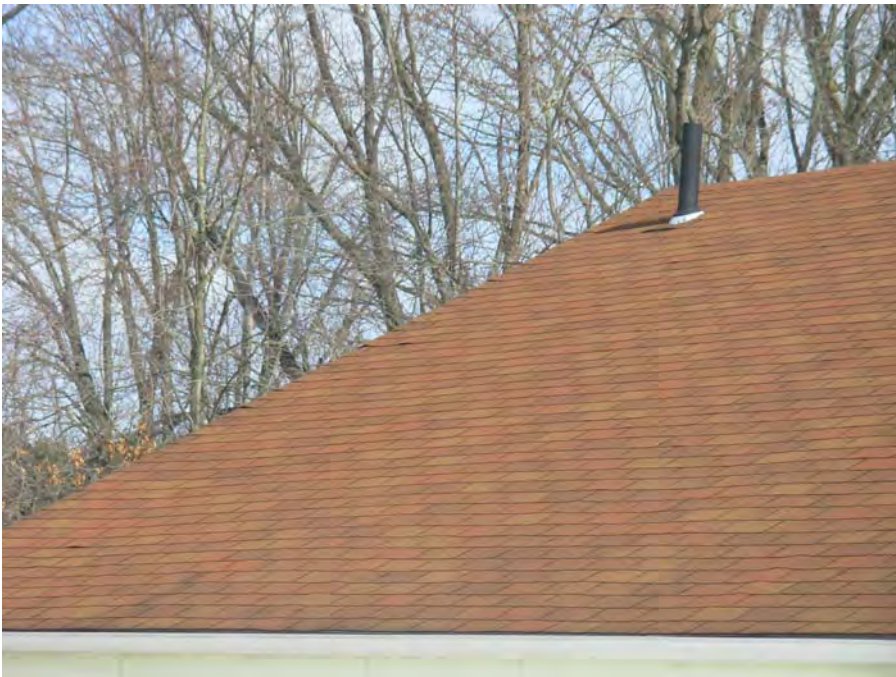
9. Spot lifting of roofing shingles
