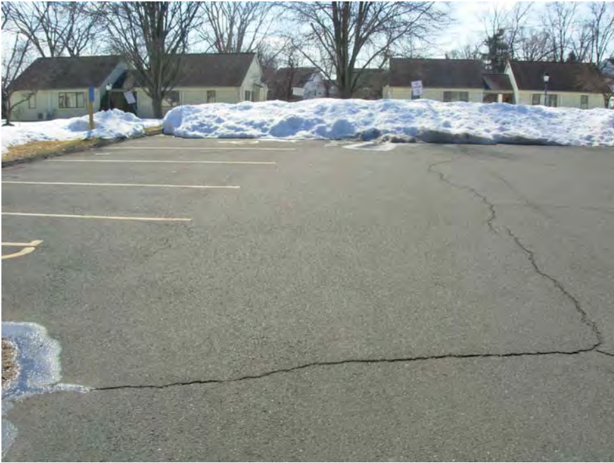
1. Sporadic cracking of parking surfaces
