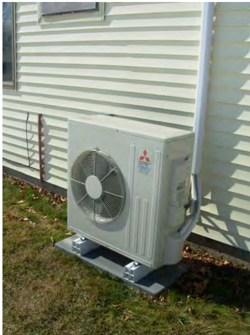
13. Typical heat pump HVAC system exterior condenser unit
